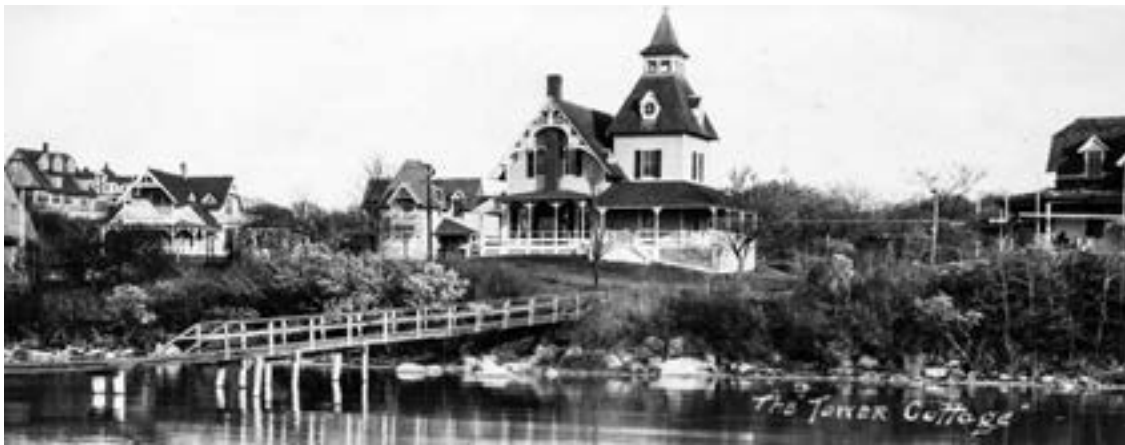
Bartlett Cottages with Tower Cottage at center (today Tapscott), circa 1920.
