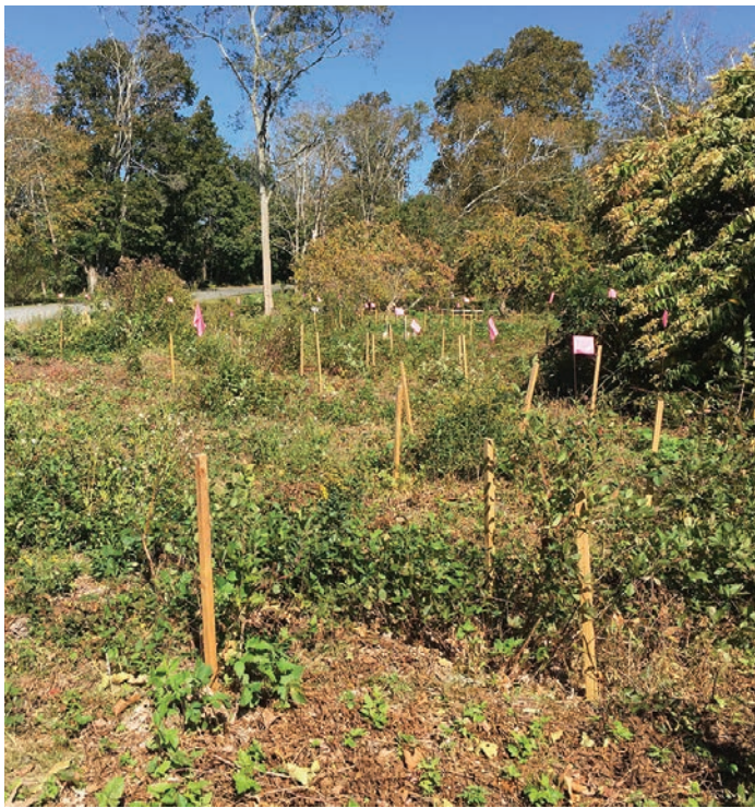
Stakes marking locations of native plantings. Photo by Jack Schneider.
