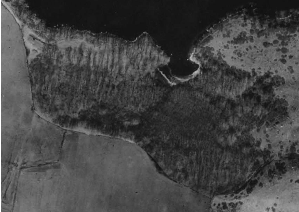
Figure 83. Millers Point (Parcel 11) and Parcel 9 wetland mid-1920s.
