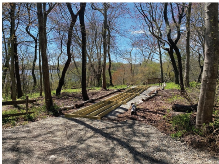
Handicapped-accessible ramp under construction at head of Treasure Pond Trail overlooking Middle Farms Pond. Photo by Bob Miller.
