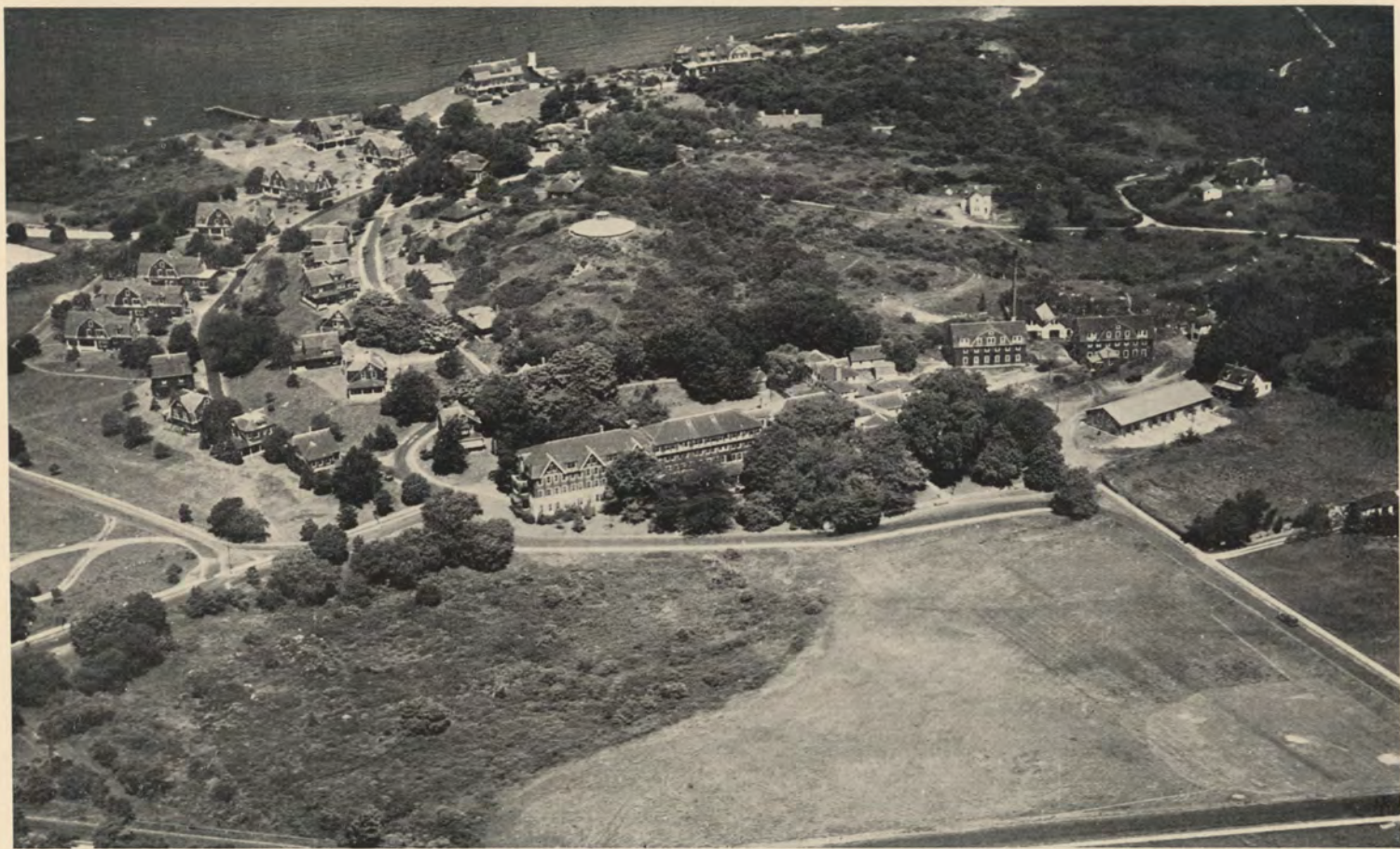
AIRPLANE VIEW OF MANSION HOUSE AND COTTAGES
