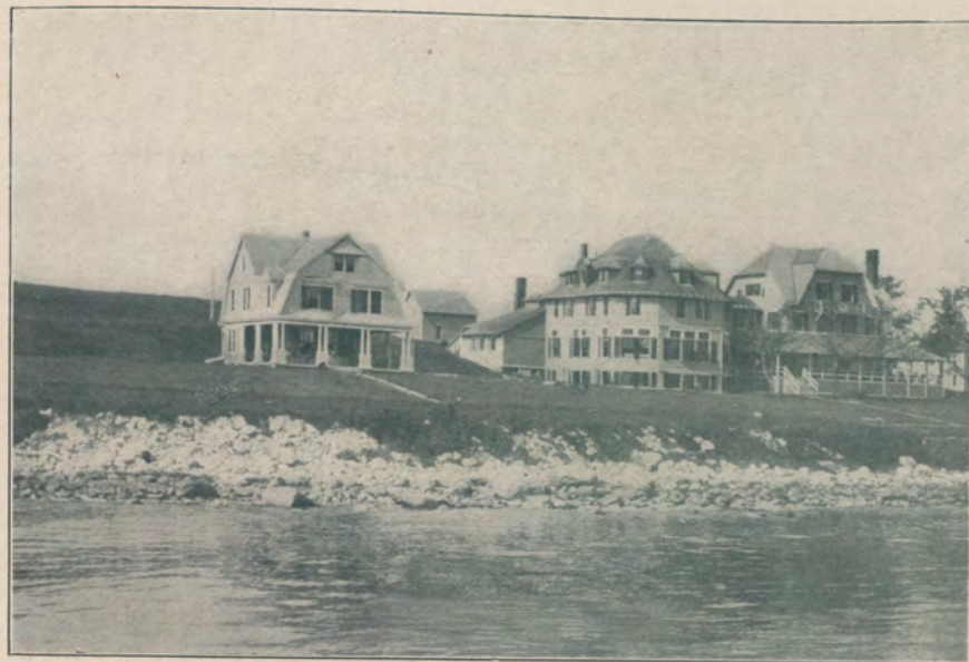
MUNNATAWKET HOTEL AND ANNEX
