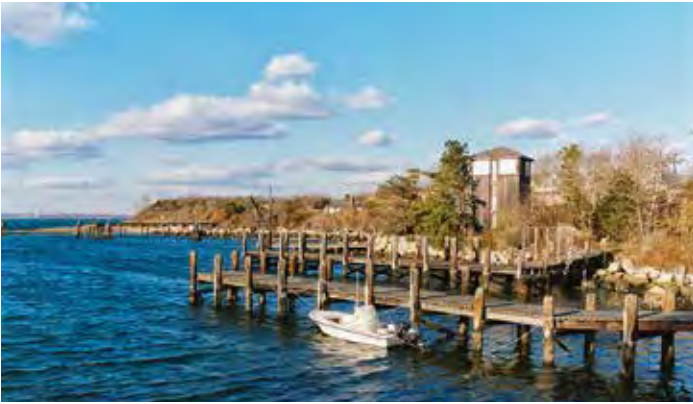
Docks on Silver Eel Cove with Pump House in background, circa 2001.
