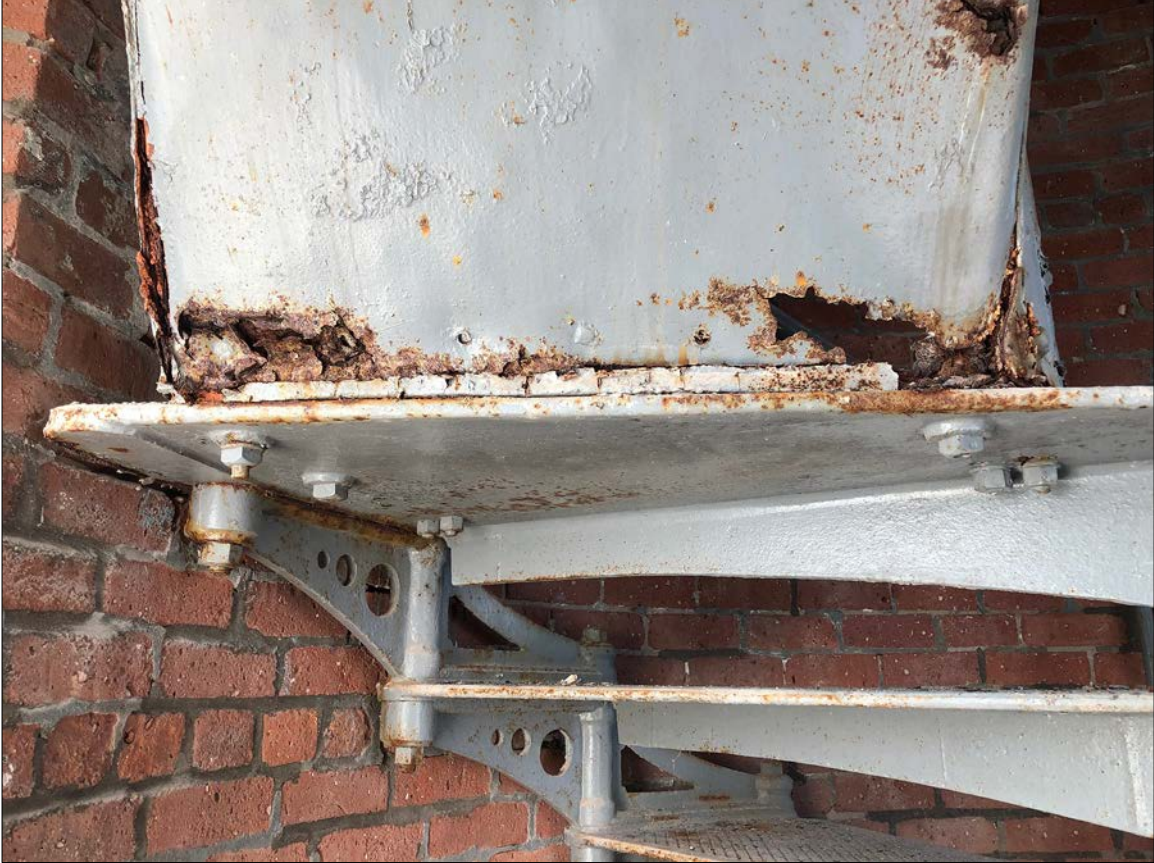
Photo 23. Just beneath the Lantern Level, the final stair run is permeated with rust resulting from water ingress above as well as deposition of condensation from being closed for long periods. Despite its appearance, damage such as this remains very restorable.
