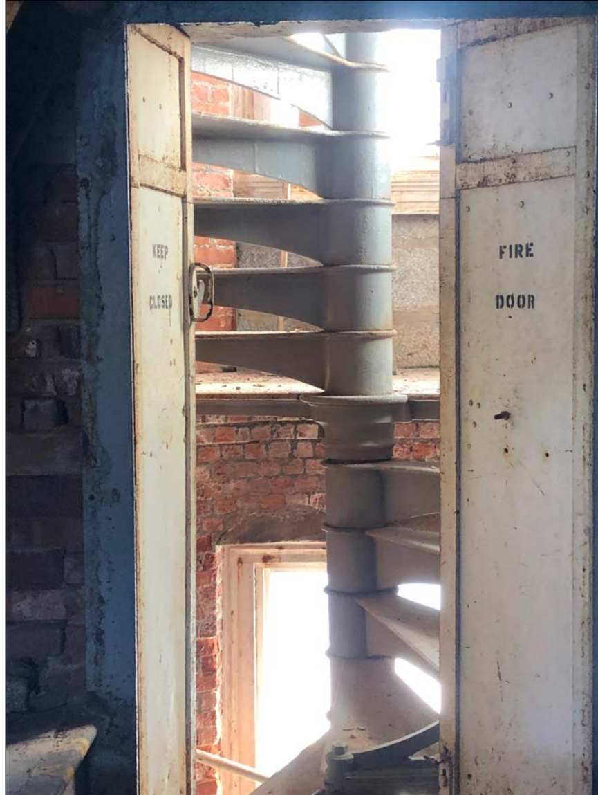
Photo 22. Cast iron spiral stairs continue directly to the Lantern, via the attic and Service Level of the Lighthouse. Water seeping through the Lantern's cast iron elements is evident throughout.
