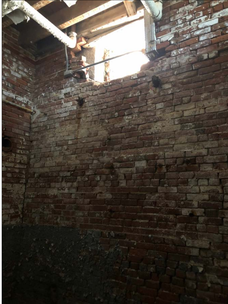
Photo 18. The cellar level within the Drum housed a variety of functions critical to Keeper & family, primarily related to food, water and heating. It is punctuated with upper windows at the level of the Drum deck for ventilation and light. Efflorescence of embedded salts is evident in the brick walls.
