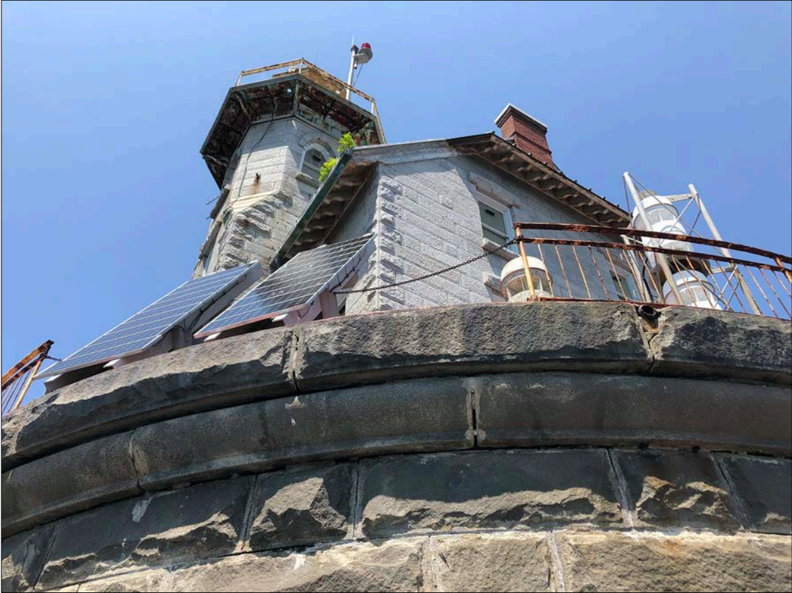
Photo 6. Missing rails, open masonry joints, gutters filled with organic matter, and similar myriad but addressable issues combine to undermine stability, even of structures built to last hundreds of years or more.
