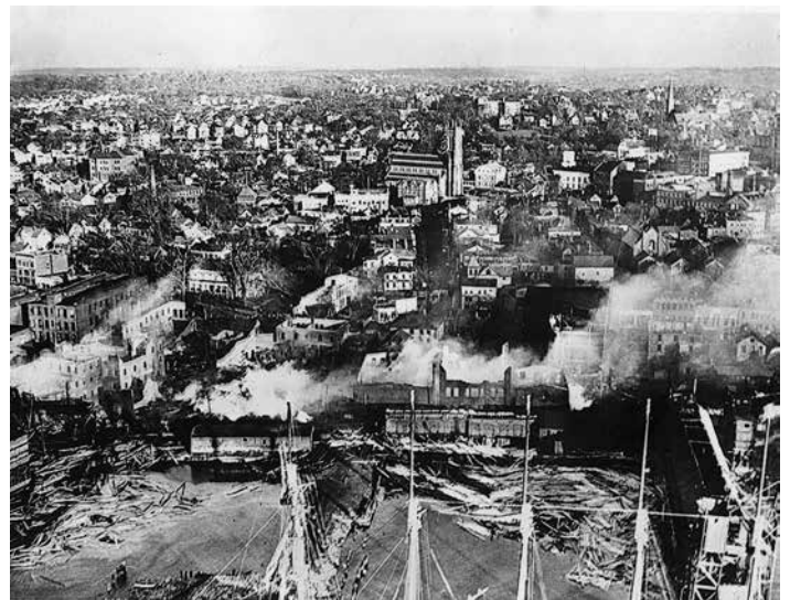
New London's Bank Street smoldering after 1938 Hurricane. News photo. Museum acquisition.
